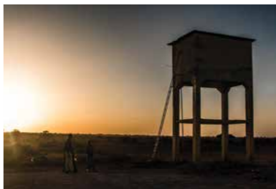
Building water tank provides sustainability for income-generating projects in drought-stricken Somalia. Image: IR Canada
