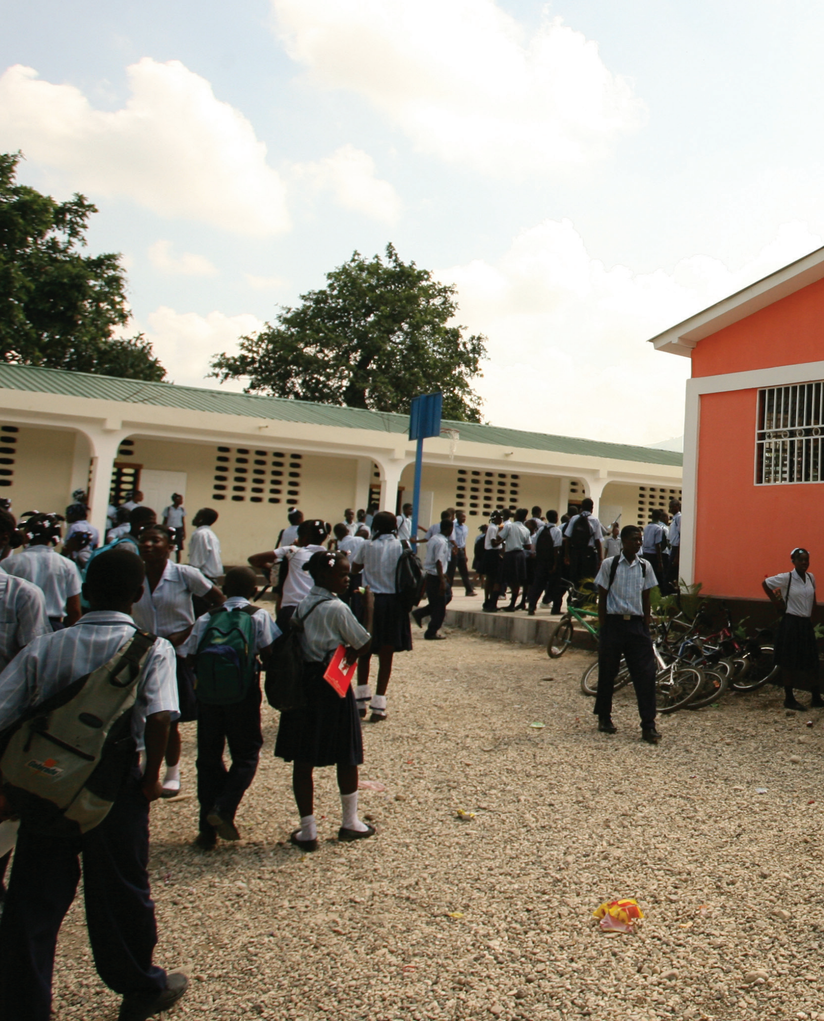
Photo: Newly constructed Lycee Dumay school provides education access to over 1,100 children. Construction of another five schools will begin in 2012.
